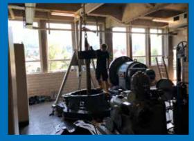
Maneuvering an old gearbox and generator out of a 1950s hydroelectric plant and bringing in a new Permanent Magnet generator called for an innovative transport and handling solution.
