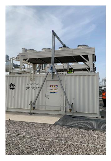
Eurosafe Solutions supplied Conrad Energy with a REID **PORTA**GANTRY which is enabling the Independent Power Producer (IPP) to comply with all the relevant working at height regulations at its Red Scar fast response power project near Preston.
